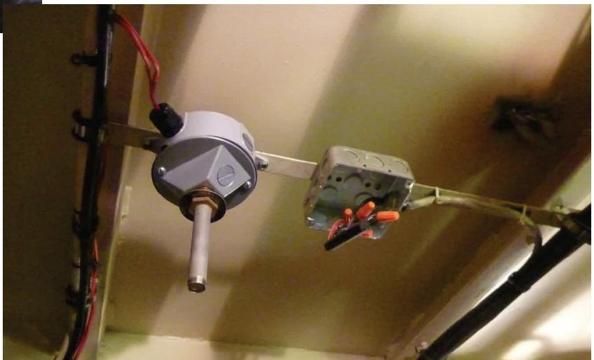
In case the picture doesn't show it very well (I couldn't really find a good angle for this shot) these five wires all terminate into a .... Bunch of wire caps. The cover to the junction box was 'not present' prior to my arrival.....
