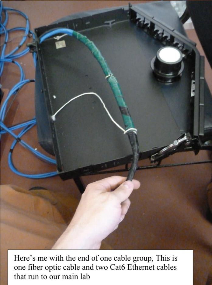
Here's me with the end of one cable group, This is one fiber optic cable and two Cat6 Ethernet cables that run to our main lab
