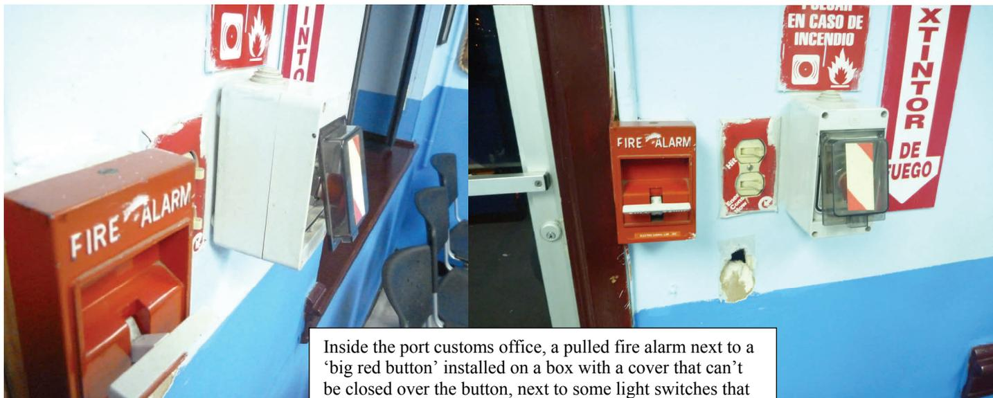
Inside the port customs office, a pulled fire alarm next to a ‘big red button’ installed on a box with a cover that can’t be closed over the button, next to some light switches that appear to be actual alarms, over a spot where someone seems to have lost interest while installing something else... probably another non-functional alarm...
