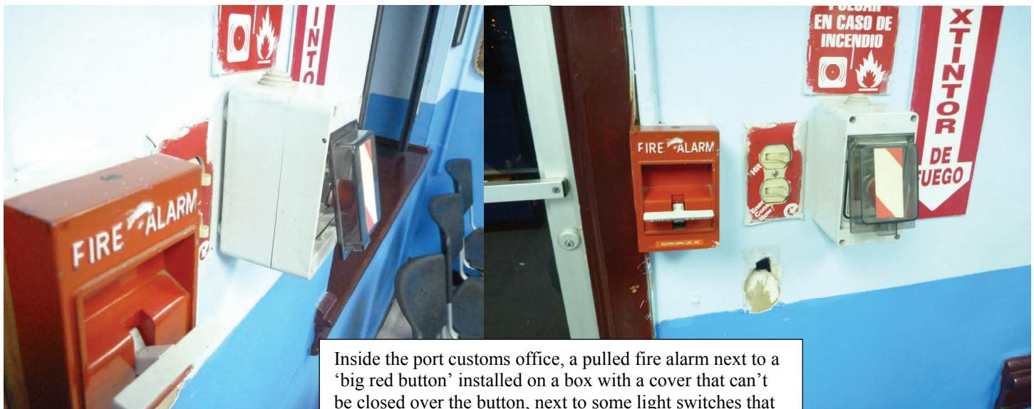
Inside the port customs office, a pulled fire alarm next to a ‘big red button’ installed on a box with a cover that can’t be closed over the button, next to some light switches that appear to be actual alarms, over a spot where someone seems to have lost interest while installing something else... probably another non-functional alarm...
